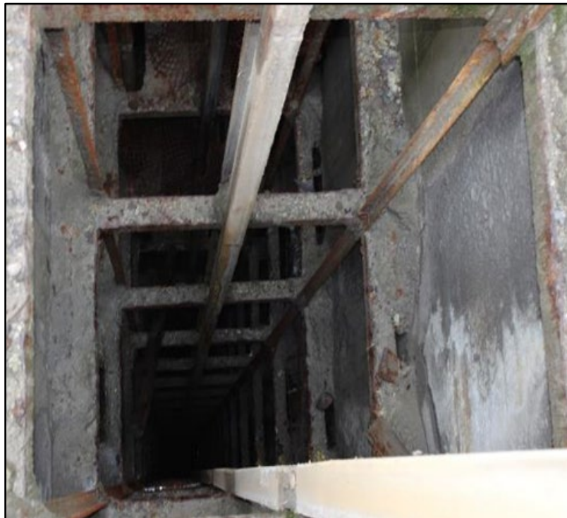
Photo 6-3: Looking down the three-compartment Santander Shaft
