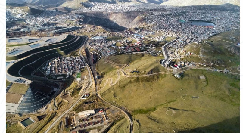
Excelsior Stockpile & Cerro De Pasco Pit
